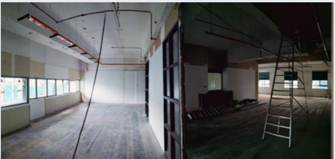
*Top Photo:* Renovation works at the studio on Level 3. The frames for the acoustic walls and the suspension for the acoustic ceiling have been installed.
